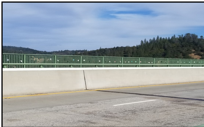
Foresthill Bridge with notes attached
